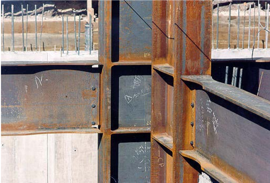
Figure 1. Reduced Beam Section (AISC Seismic Design Module (2007))
